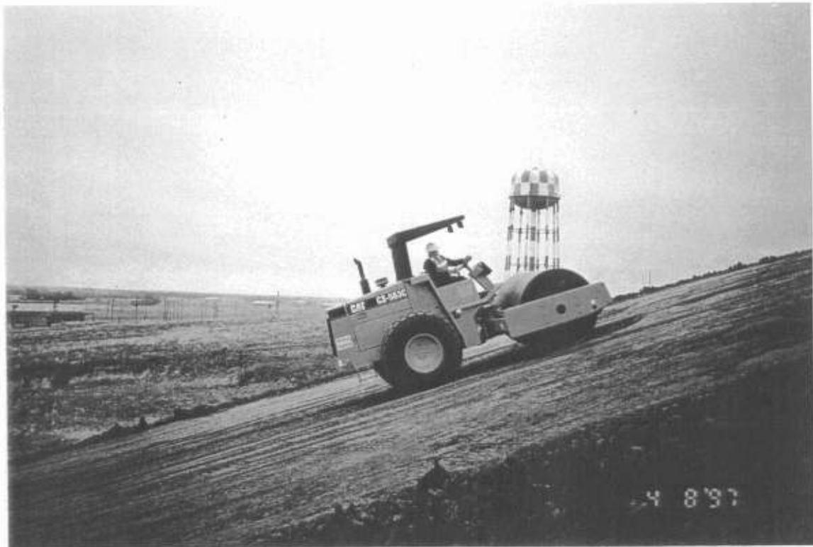
Photo No. 15 Smooth drum rolling the test fill surface.
