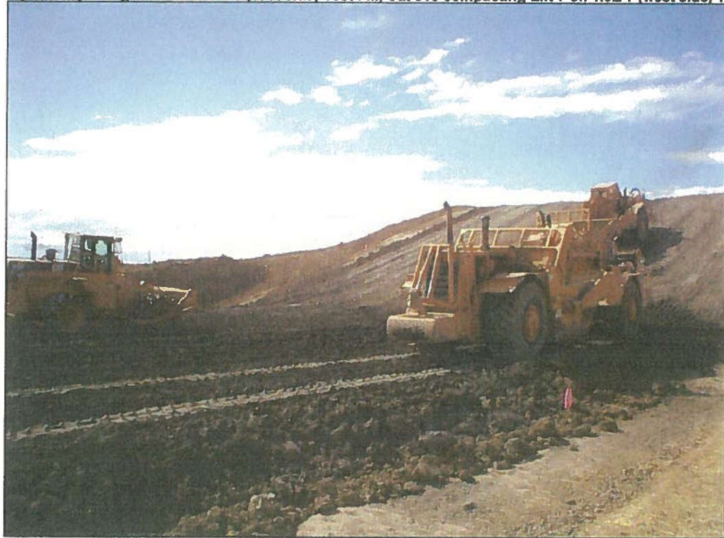
6 - Cat scraper compacting lift 6 on 1.0xE-8 (east side) Test Fill, Cat 815 compacting Lift 7 on 1.0E-7 (west side) Test Fill
