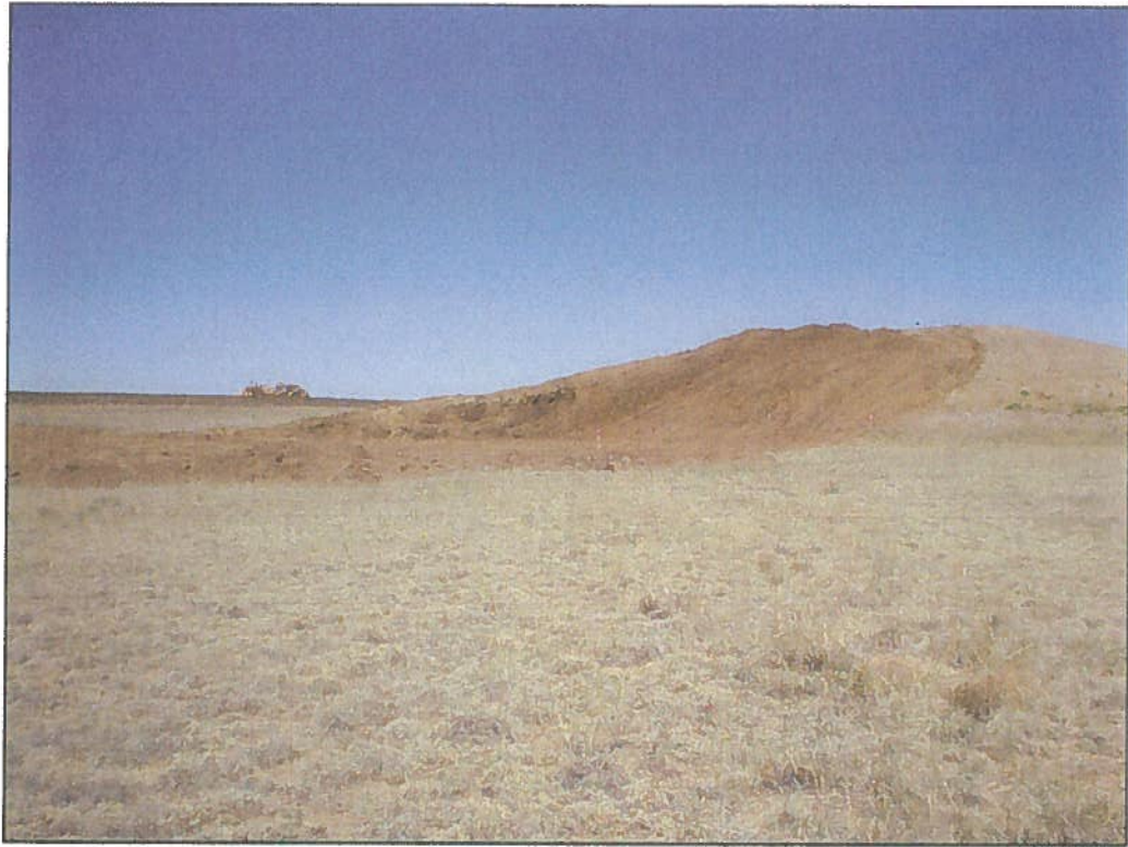
1 - Grading south end of existing stockpile for test fill pad
