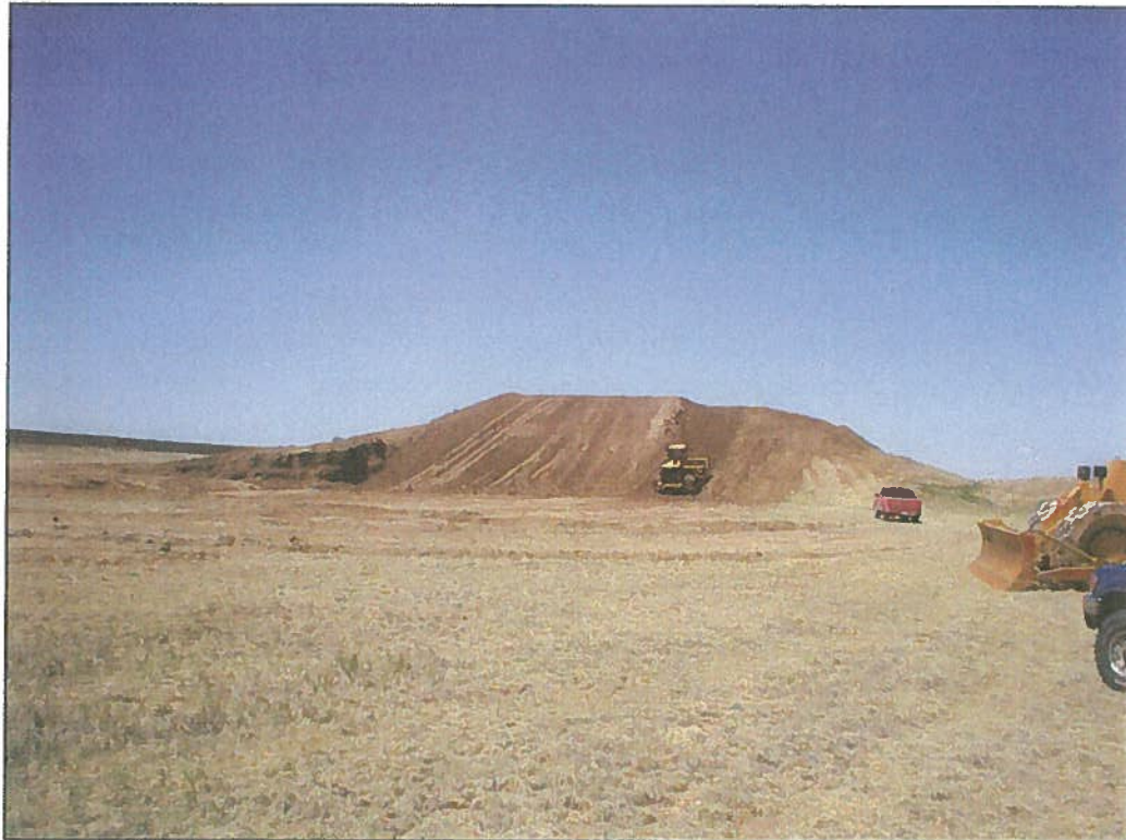
2 - Grading and compacting Test Fill subgrade
