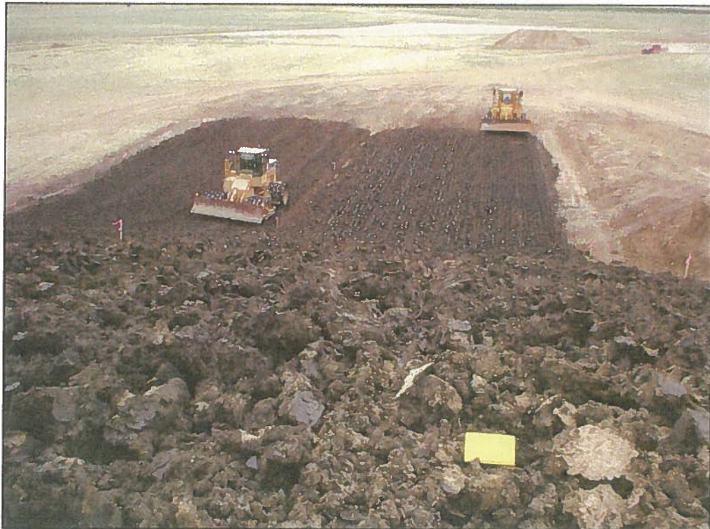
4 - Cat 815 (east side - left), Cat 825 (west side - right) compacting clay
